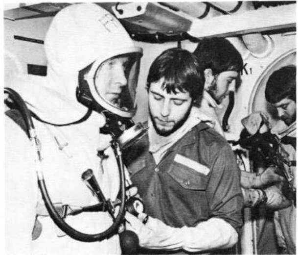
Two of the damage control team on *Invincible* check their fire-fighting suits and breathing apparatus, ready for action. The fire and smoke hazard was shown to be a major contributory cause to ship losses suffered by the Task Force. Toxic fumes given off by plastic materials used for furnishings and wall coverings sometimes prevented teams from reaching the real seat of the fire. (MoD)
