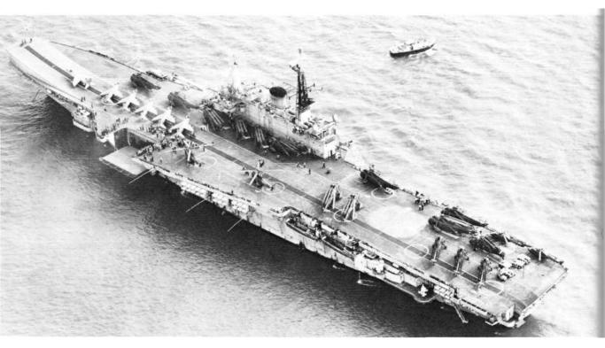
HMS Hermes, flagship of the Task Force, on her return to the UK. On deck can be seen various aircraft which took part in 'Corporate'. Forard are six Sea Harriers, and six Sea King HAS.5 ASW helicopters of N0.826 NAS; at positions 3 and 4 are two RAF Pumas; at 5 and 6 are two more HAS.5 Sea Kings, and a Commando Sea King HC.4 of N0.846; and right aft are an HAS.5 and an HC.4, four Wessex and two Lynx. (C. S. Taylor)
